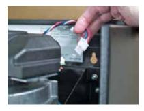
Unplugging fan control harness plug will drive the fan into manual high speed operation for vent leak test
