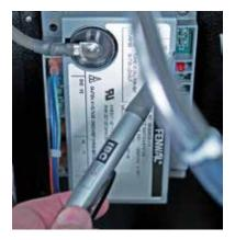
Fenwal ignition module - Microamp  $(\mu A)$  test points are shown at top right corner of module (above red L.E.D.)
