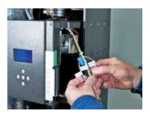
Line voltage leads for power supply, primary pump and variable speed output
